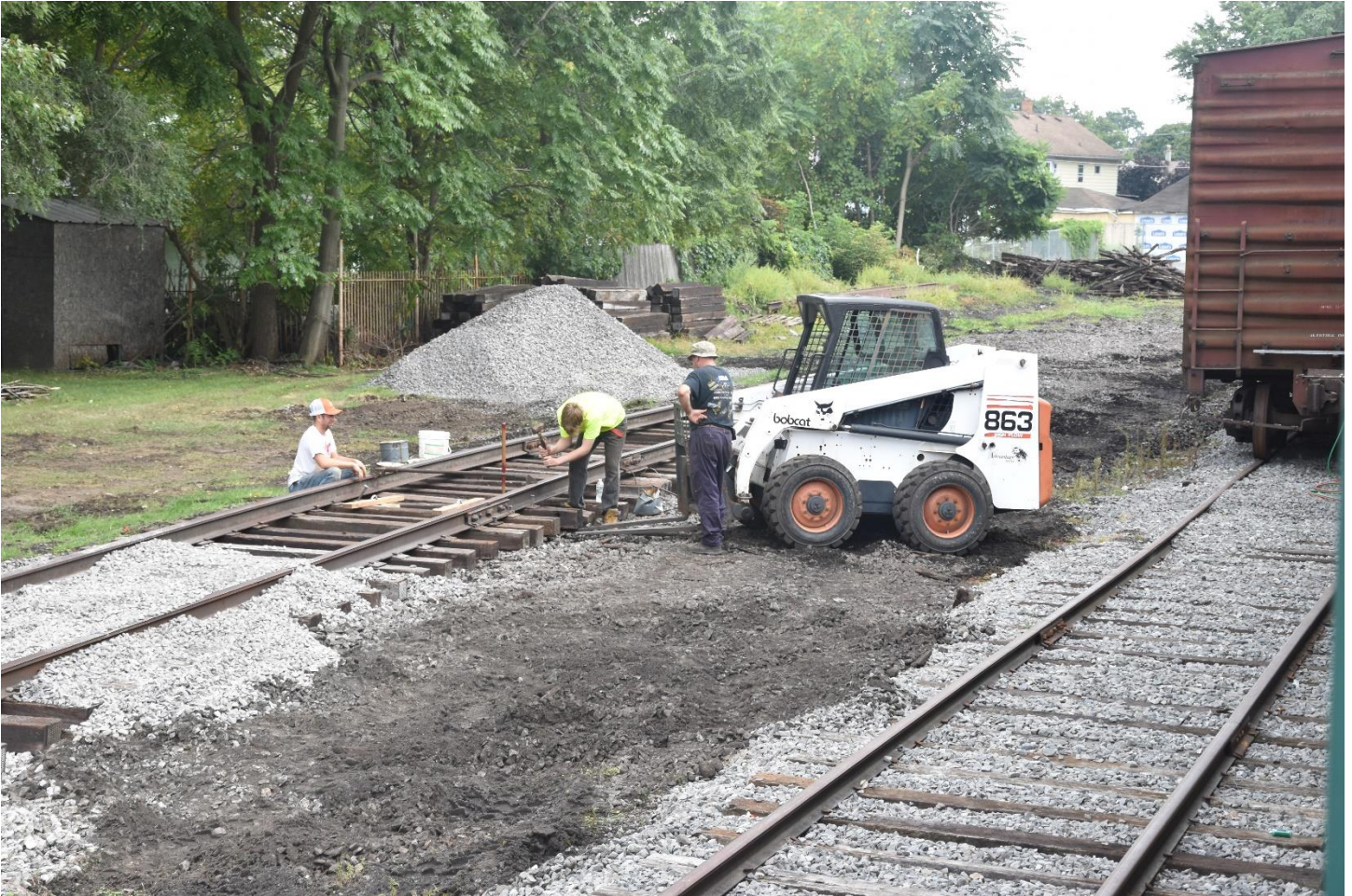
All photos trackwork project by Jim Ball
