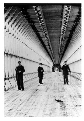
Left: This photo shows the interior of the lower level of the bridge. This was a wagon / carriageway path. Above are the railway tracks. Imagine what it must have been like crossing this bridge with its creaking timbers and vibration noises caused by moving trains!
