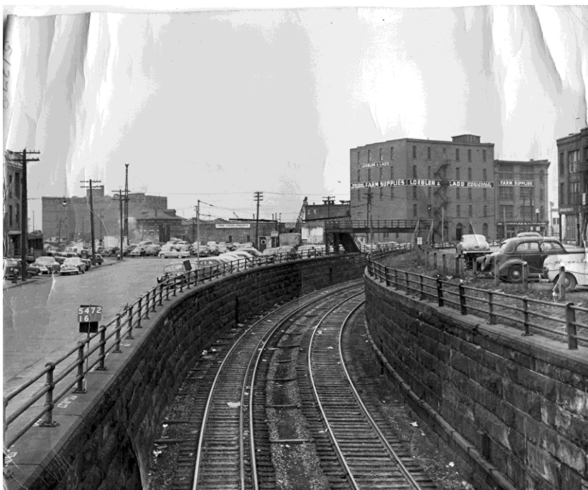
A general view of the Terrace right of way. The grade was fairly steep, and the curves were tight from Exchange Street station up to street level. The track was relocated south to the abandoned bed of the old Erie Canal in the early 1950s and this cut has been covered over and today is unidentifiable, being beneath the viaducts of Interstate 190. This view looks west, from around where Main Street crossed the line. Niagara Frontier Chapter, NRHS archives
